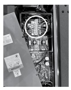
Remove terminal box lid and locate P1 & P2 for connecting the pump control relay and terminal 5 & 6 for connecting external automation heater control.
